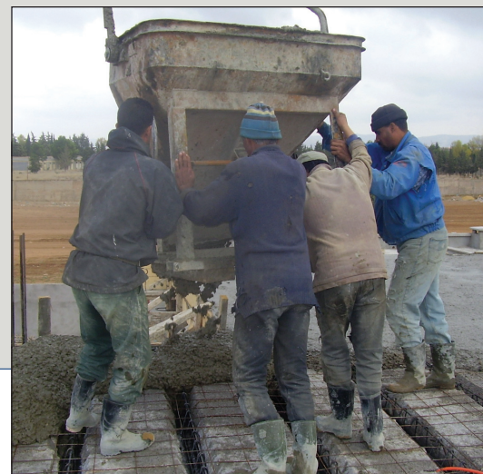
Above: Site batching is the norm in Algeria because ready-mix is not available. Above, right: Concrete is batched at a construction site in Algeria. Right: Site batched concrete has a 4-inch slump with strength of 3500 psi.
