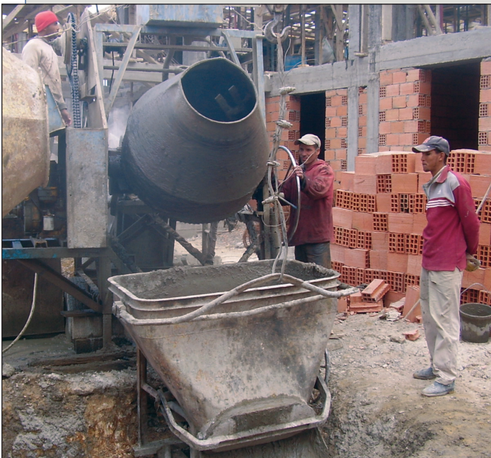
Above: Site batching is the norm in Algeria because ready-mix is not available. Above, right: Concrete is batched at a construction site in Algeria. Right: Site batched concrete has a 4-inch slump with strength of 3500 psi.
