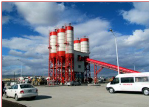
The Premium Concrete batch plant located in Ulaanbaatar plans to seek the National Ready Mixed Concrete Certification.
