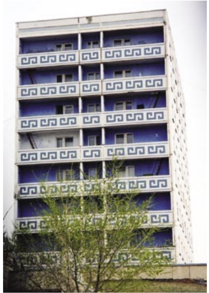
This functional apartment building, of rectilinear design and with decoratively painted exterior elements, is formed from accelerated-cure precast concrete. The precast was supplied by a plant in Ulaanbaatar, Mongolia's capital, a city of 600,000 and some 10 mi. (16 km) distant. The capital city has four precast plants
