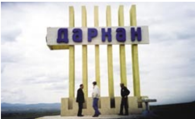
Mongolian cities erect these entranceways or gates. This one on the outskirts of Darkhan is formed from painted precast elevated elements supported upon a cast-in-place base
