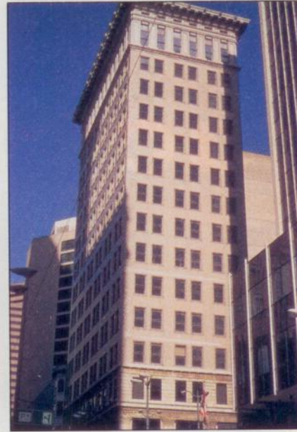
The first high-rise reinforced concrete skyscraper in the United States was built in Cincinnati, Ohio. This 16-story building was constructed in 1902 by Fero-Concrete Construction Company. It was built at a time when no buildings with more than 6 stories had been constructed of reinforced concrete. The building is still in use.
