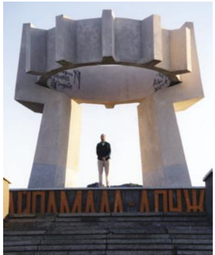
Within the industrial city of Erdenet stands this tribute to the friendship between Mongolia and the former Soviet Union, which existed at the time of its construction. The precast concrete elements shown represent two hands holding aloft a manufactured gear, symbolizing both nations working together toward common economic goals
