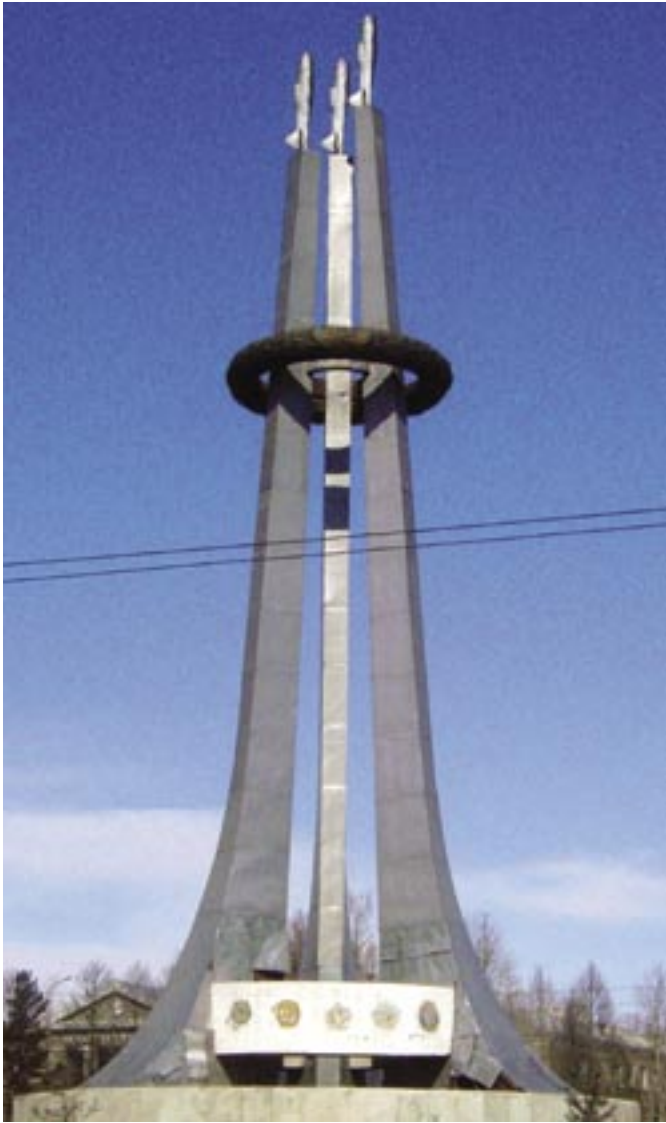
Near the center of the Mongolian capital city is this Air Force Memorial, a tribute to Mongolian airmen who served in World War II. Shapely curved and vertical precast elements and other segments are supported on a cast-in-place foundation
