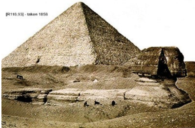
This photo of the pyramids at Giza taken in 1858 shows the white gypsum mortar between the blocks.
