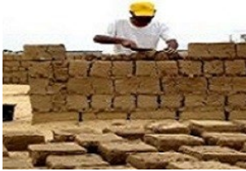
Building a wall with sun dried brick and mud mortar.
